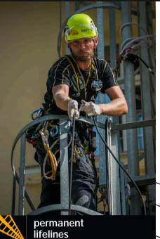
Permanent lifelines serve to secure workers in places where it is possible to set up fixed anchor point in the working place or near it. These are then interconnected by steel rope or a rail. For moving and securing, the worker uses connectors (EN 362) or special slider made for this purpose and supplied by the system manufacturer. The advantage of permanent lifelines is their long operating life and variability of use.
